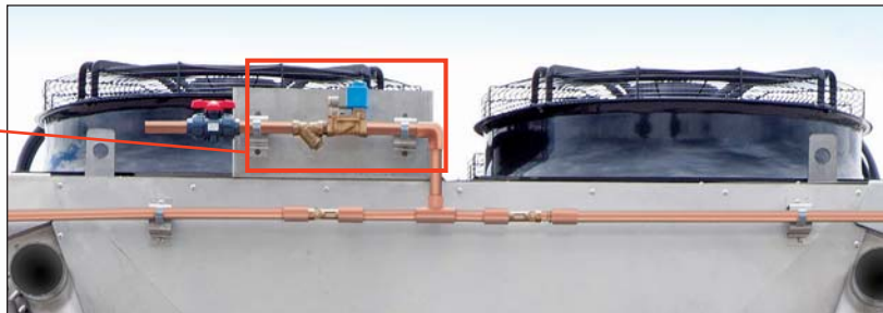
Water supply solenoid valve arrangement
