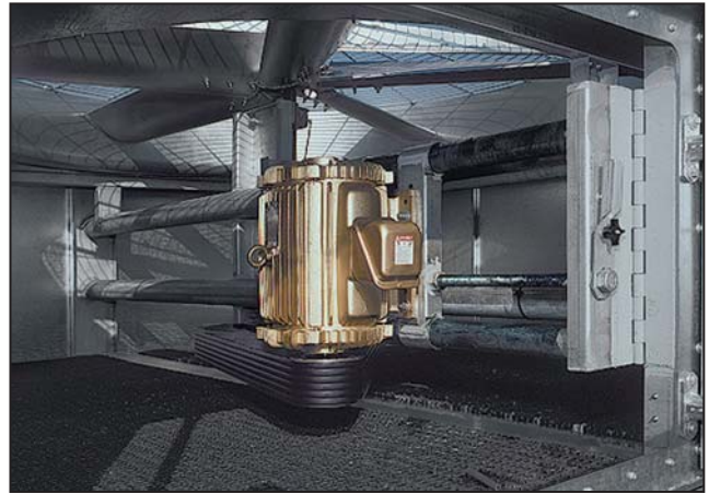
Motor Base Assembly
